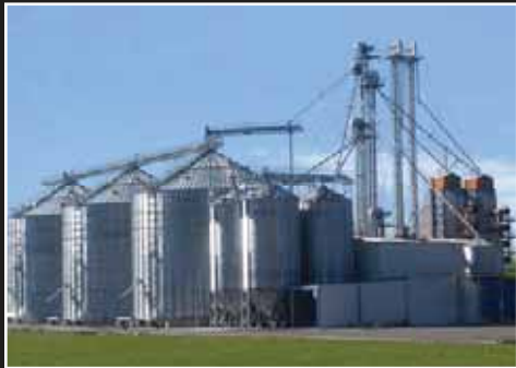
SCAFCO Bins located in Chile
