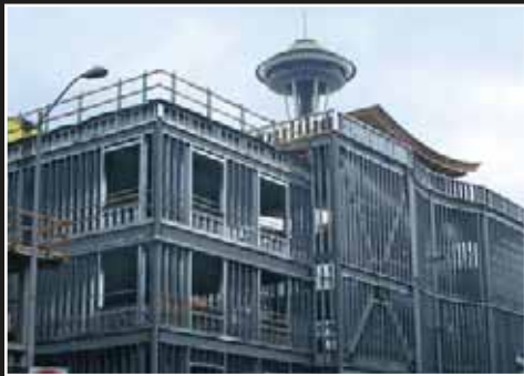
Stud Framing Project in Seattle, WA
