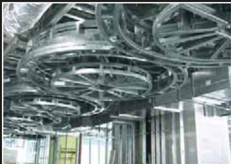
Radius Soffits Project in Sacramento, CA
