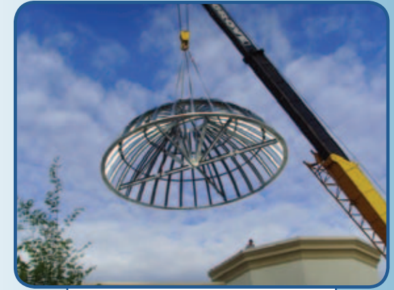
EXTERIOR ROOF DOMES
